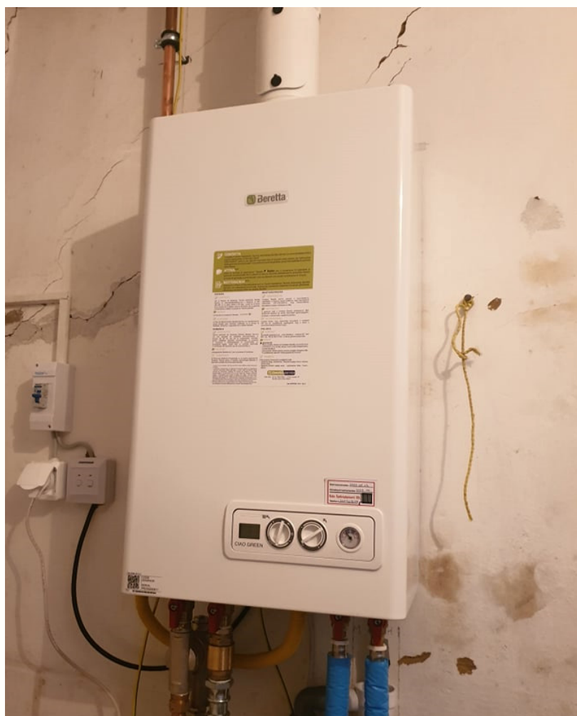
After: New boiler and central heating (Magyarnándor, Nógrád county)
