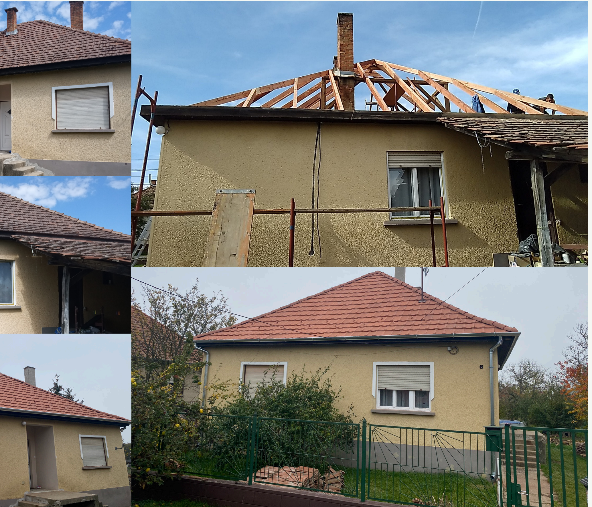
Before and after complete roof reconstruction (Magyarnándor, Nógrád county)
